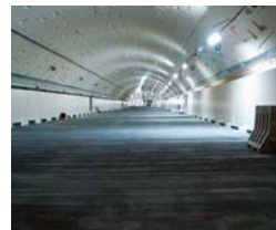
SMART Tunnel Kuala Lumpur, Malaysia
