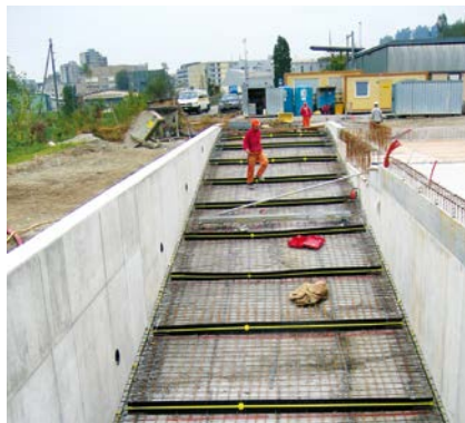
Preventive waterproofing at construction joints, crack control (dummy) joints and penetrations
