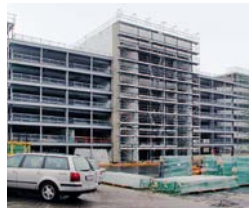
Airport Munich, Germany
