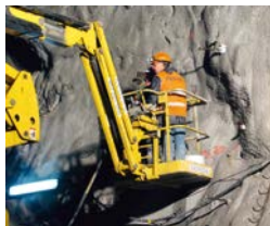
High speed train track Udalaitz, Spain
