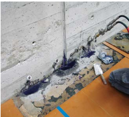
Remedial waterproofing
