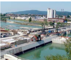
Power station by the river, Rheinfelden, Switzerland
